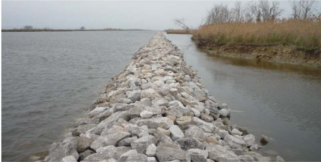
Figure 35: Constructed breakwater along the GIWW in Jefferson County, TX (Ducks Unlimited, 2013)
